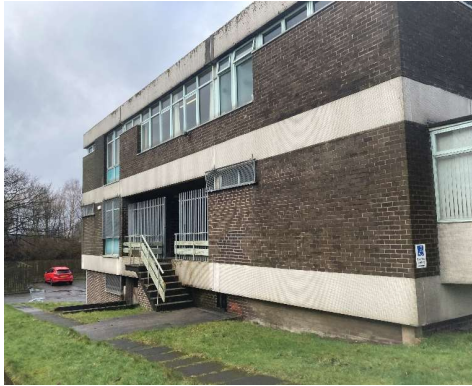
Form of Construction Photo 1 Concrete frame with brick infill, aluminium single glaze windows to the buildings side and rear
