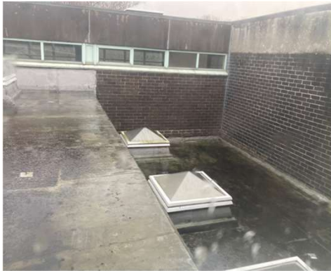
Form of Construction Photo 4 Single-ply membrane roof weather covering
