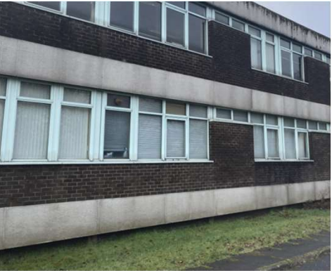
Form of Construction Photo 2 Concrete frame with brick infill, uPVC double glaze windows to the building's front elevation
