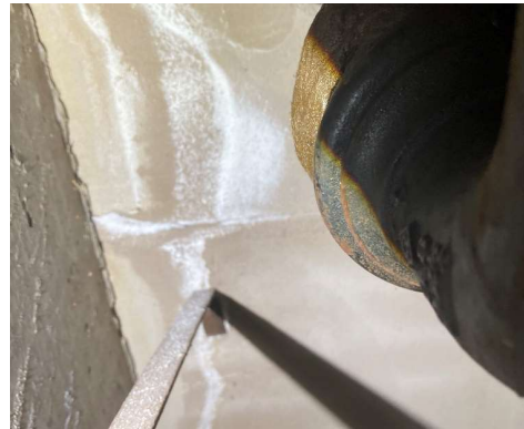
RAAC Observation Photo 3 Penetration through slab, evidence of water ingress at slab edge
