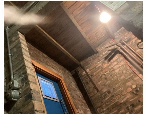
Form of Construction Photo 8 Lift motor room, Timber structure and timber roof deck
