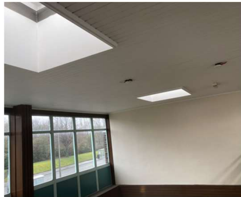
Form of Construction Photo 6 Shiplap cladding ceiling finish
