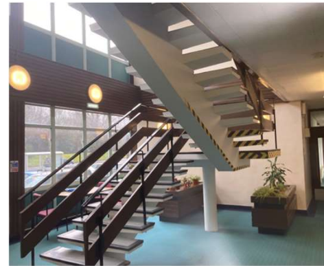
Form of Construction Photo 5 Concrete internal stairs at main entrance
