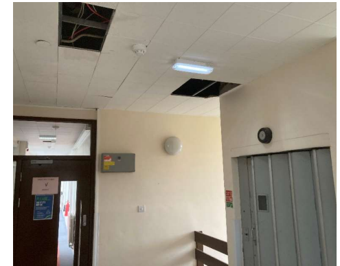
Form of Construction Photo 7 Suspended ceiling finish with concealed grid system
