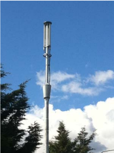
The photograph below shows newly installed streetworks pole with shroud removed. It is clear that there is space for 2 banks of antennae
