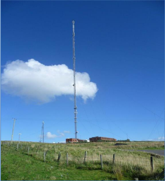
Main TV broadcast Mast (305m)
